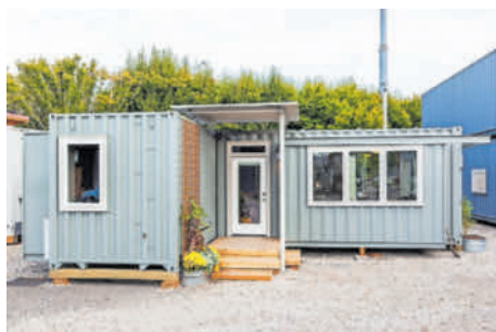
Carl Coffman of Relevant Buildings turns shipping containers into homes that are affordable, UBC compliant and sustainable. Home Builders Association of Metro Portland
